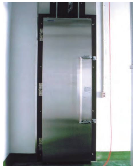
懸肉用片開扉 Single-leaf swinging door for meat hanging chambers
