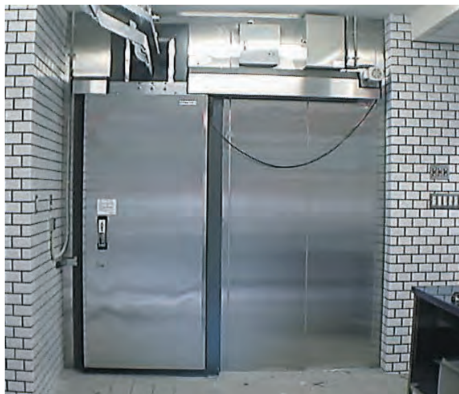
懸肉用電動片引扉 Motorized single-leaf sliding door for meat hanging chambers
